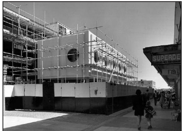
■ The Advice Centre under construction in 1977.
